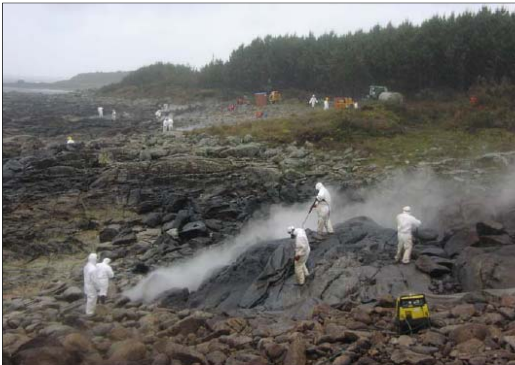
Figure 12: High pressure washing of tidal zones with hot water, © ITO PF
