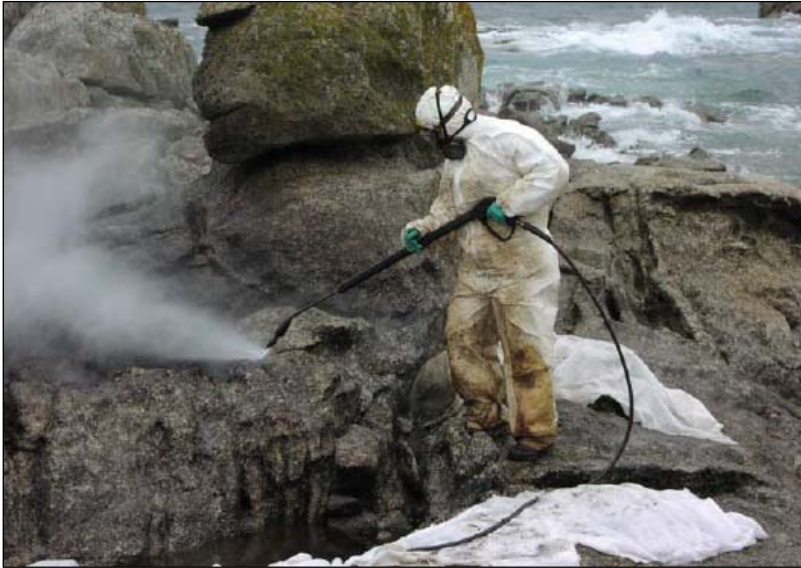
Figure 10: Hot water washing of oiled rocks, © ITO PF
