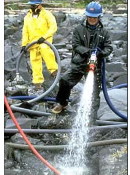
Figure 11: High Pressure washing
