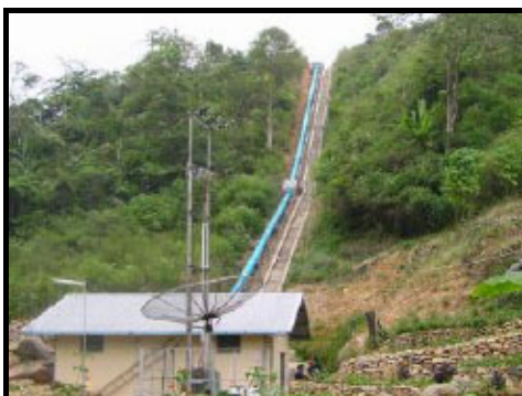
Figure 21: Penstock, source: GTZ
